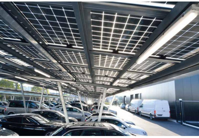
Photovoltaic carports have been installed in the new Wondercar bodywork building in Drogenbos. The produced electricity reaches 301 MWh per year, allowing to recharge between 50 and 100 VW e-Golf or almost 150 Audi Q7 e-tron a day.
